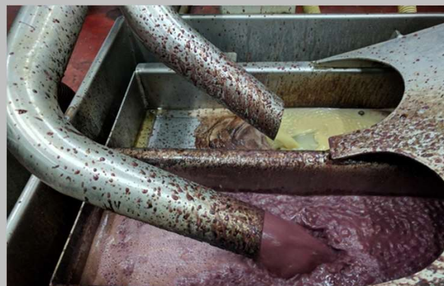
Fig. 1. Local council 'Zemer', Israel, with a three phase extraction system
